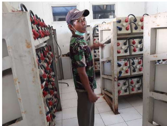
Fig. 7. Technical Personnel on Tunda Island
